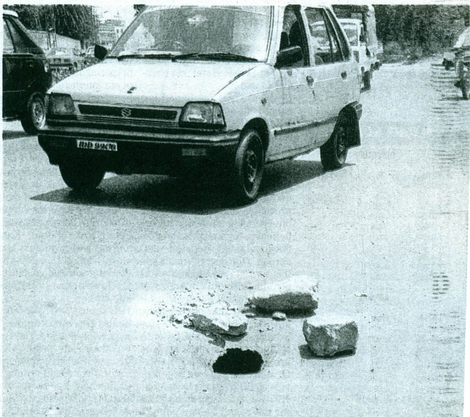
RAWALPINDI: Someone has placed stones around a hole on Liaquat Road near Tehsil Municipal Administration Office to warn motorists and pedestrians. — Sardar Heera
